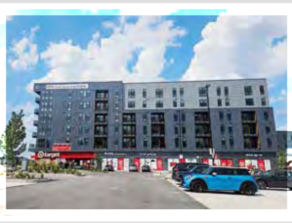
The new Target store is located along Grand Boulevard between Gratiot and Papin streets.
